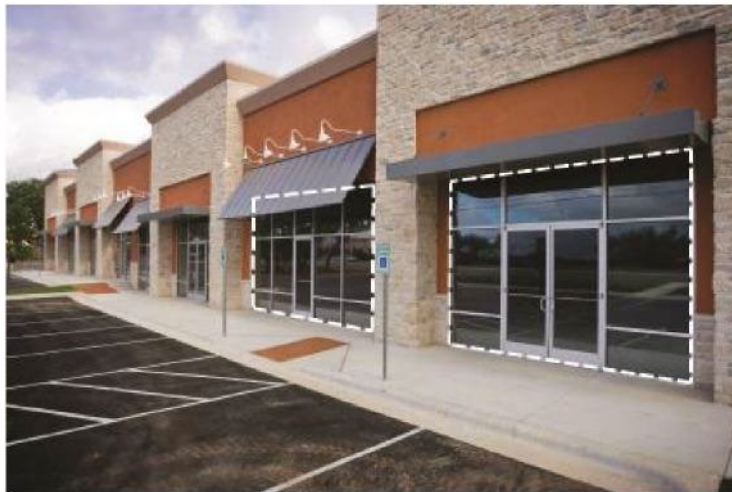
Figure 1117-K: The window area is illustrated within the dashed line area for the two storefronts in the above image. The dashed lines highlight two separate window areas due to the separation by an architectural feature not related to the windows.
