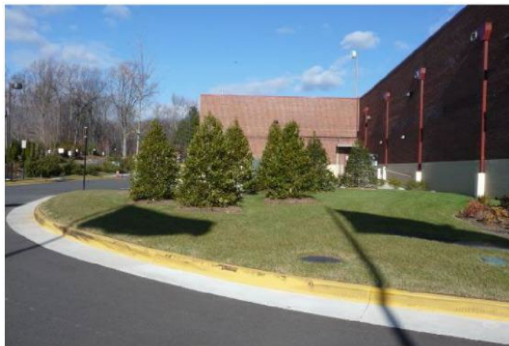
Figure 1113-A: The above image illustrates a vegetative screen that hides HVAC equipment and a dumpster.
