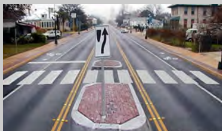
Pedestrian refuge islands are added to portions of the right of way dedicated for extended turn lanes.
