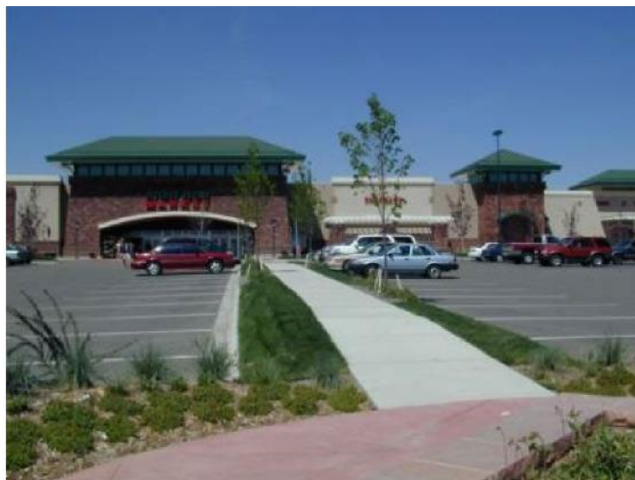
Figure 1115-E: This photograph illustrates how a sidewalk connecting the public sidewalk to the business can be integrated into the required landscaping.
