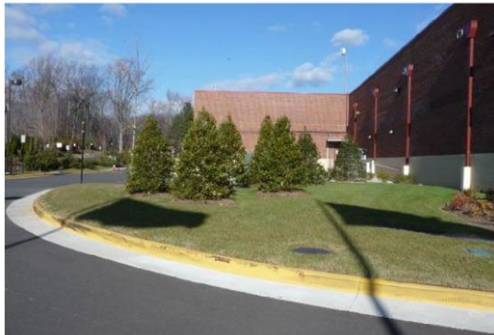
Figure 1113-A: The above image illustrates a vegetative screen that hides HVAC equipment and a dumpster.
