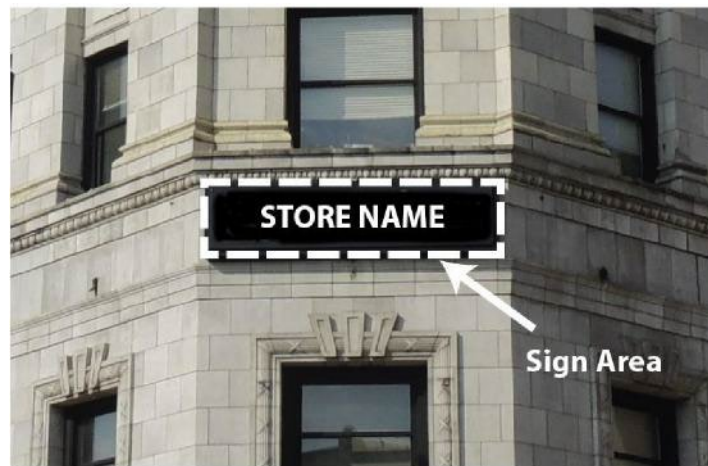
Figure 1117-C: Illustration of computing the sign area for wall signs with a background panel or cabinet.
